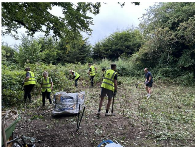
Clearing the site of the former orchard
